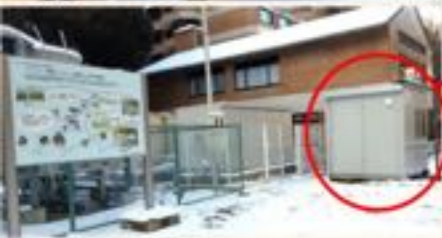
Panoramic view of the heat storage facility
